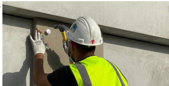
Gently hammer the pin in place
