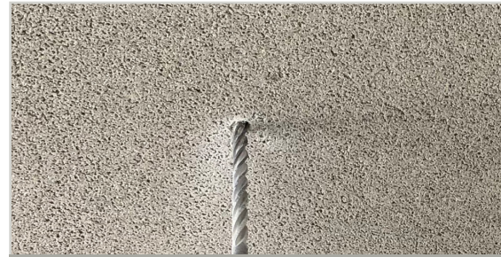
Drill into the centre of Reapor
