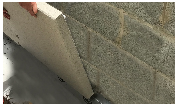
Apply the tile to the substrate with firm pressure
