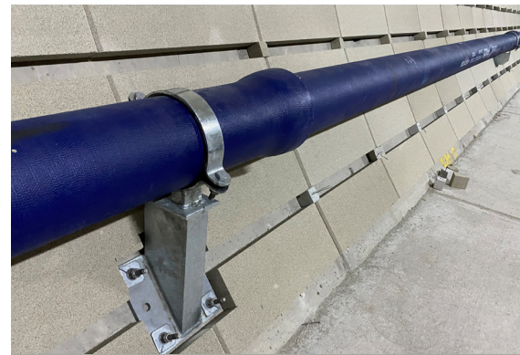
Tunnel application - Reapor installed on the wall
