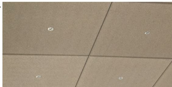
Completed overhead installation
