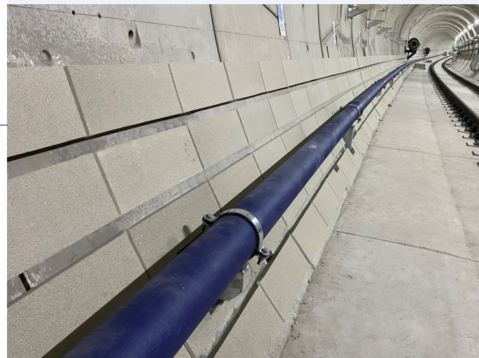
Reapor 625 x 208 panels installed in tunnel application
