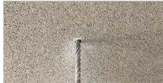
Drill into the centre of Reapor
