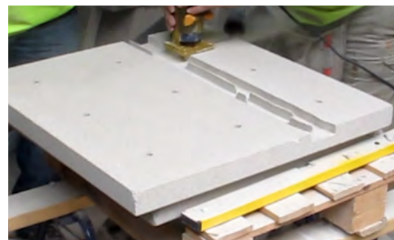
Reapor can be routed to allow cable access
