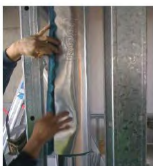
Wrap each segment with an overlap
