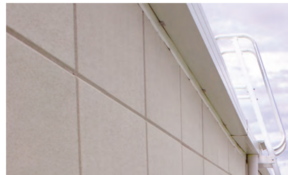
Regularly inspect flashing for functionality
