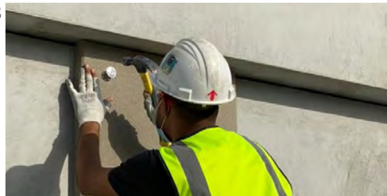
Gently hammer the pin in place
