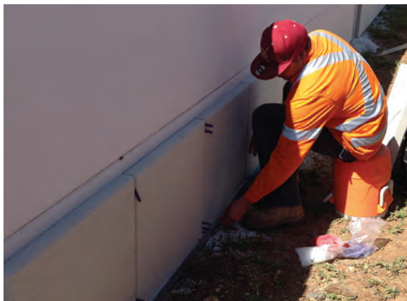
Installing Reapor on site using flexible, thixotropic adhesive.
