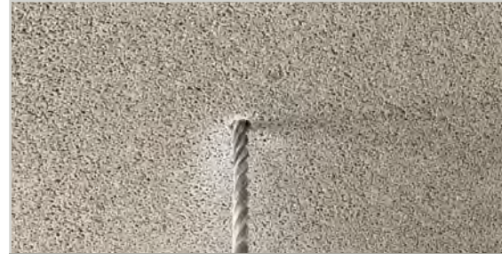
Drill into the centre of Reapor
