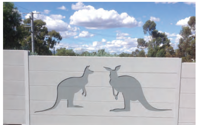
The decorative front of the Noise barrier wall (Reapor applied to reverse side)
